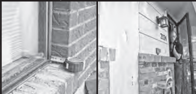
(Left) Recessed window: For hurricane protection, it's best if your windows are recessed at least 2" from the face of the wall so the shutter can be mounted inside the recess. (Right) Improvised window shutters are a great way of protecting your home against the elements and potential intruders, but if you want to use them in a disaster, you need to start working on them now.
