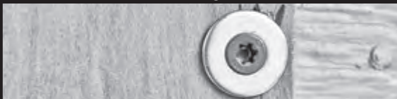
Torx: For security against looters and intruders, use non-standard screw heads for your mounting screws — like the Torx head shown here. Note the screw passes through a flat washer to increase the surface area in contact with the plywood and make prying it off more challenging.
