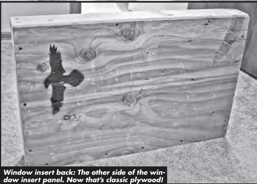
Window insert: A simple window insert can be installed from the inside to secure potential avenues of entry. The insert is made from a piece of plywood and a 2x4 frame. Note the foam insulation panel to help retain heat.
