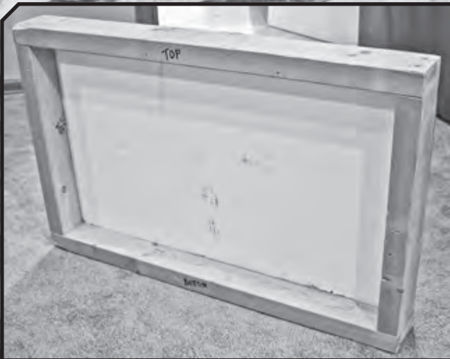
Window insert: A simple window insert can be installed from the inside to secure potential avenues of entry. The insert is made from a piece of plywood and a 2x4 frame. Note the foam insulation panel to help retain heat.
